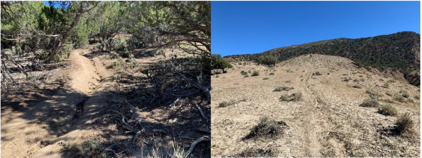
Photo 1 and Photo 2: Existing trails with lack of trail maintenance.
